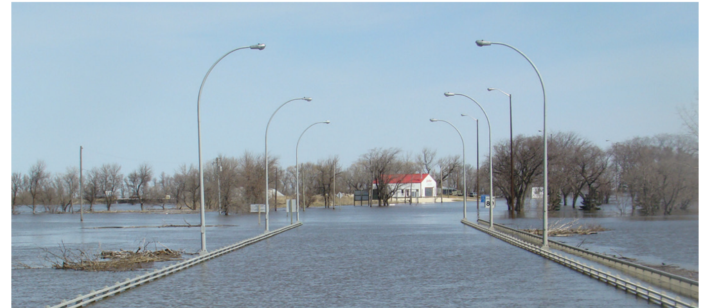
Flood water covering a bridge in the Town of Morris, Manitoba.
